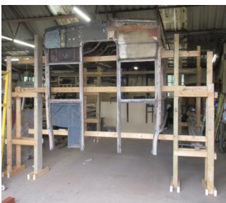
The lower saloon lifted to release the underframe.
