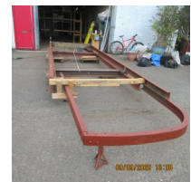
The original steel underframe after cleaning up. Sadly there has been too much corrosion and a replacement underframe will have to be made.
